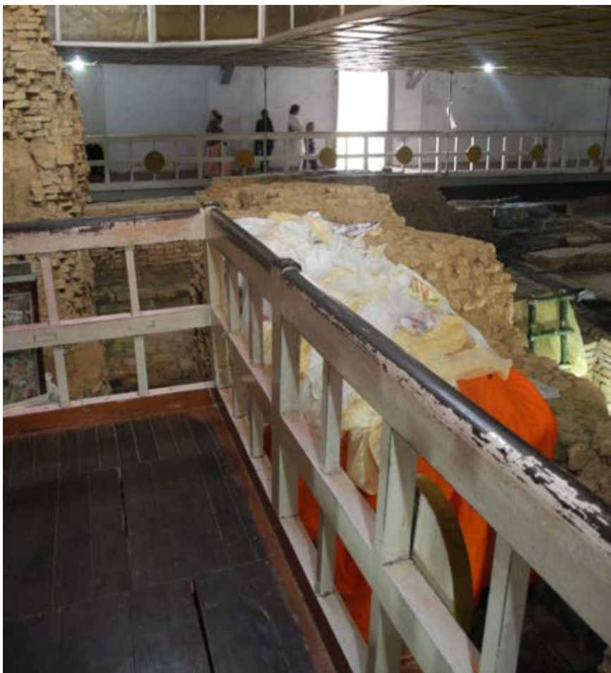
Figure 2.3 Photo showing the current walkway within the Maya Devi Temple, and brick wall to its right (eastern) side that would be removed.
