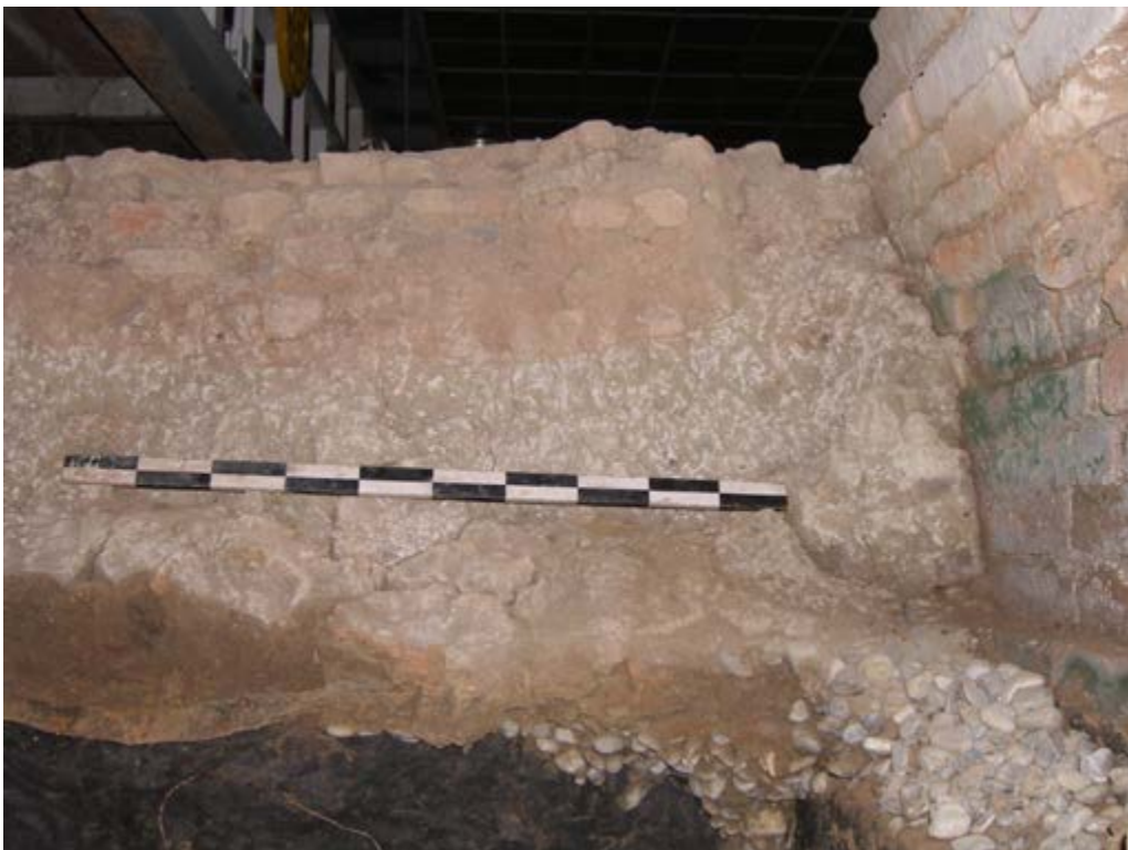
Figure 8.2. The exposed section of brickwork in Trench ENE before cleaning of the section. note also the geotextile covering the unexposed sections lower down, and part of the gravel fill to the right.
