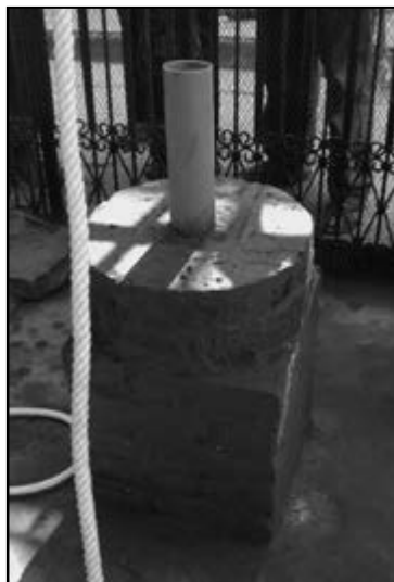
Figure 143. The new basement supporting the capital.
