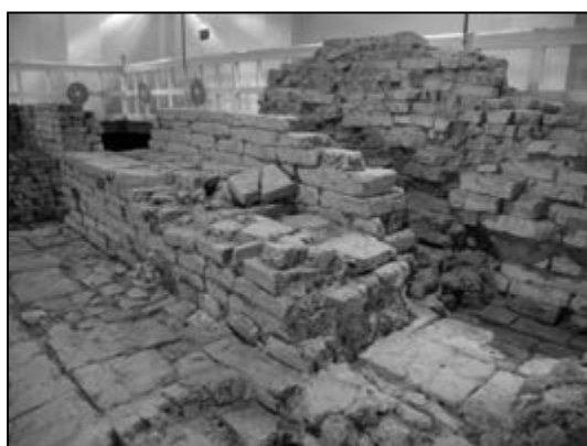
Figure 154. The wall before the restoration
