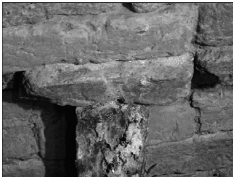
Figure 162. Gluing of broken brick with lime plaster
