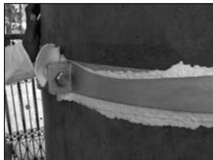
Figure 138. Applying the silicon rubber protects the stone from the iron corrosion products.
