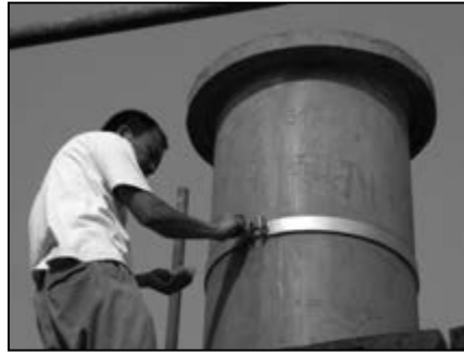
Figure 139. Finishing the belt with the varnish.
