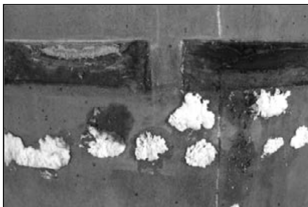
Figure 10. The surface of Pillar after the removal of the lower belt
