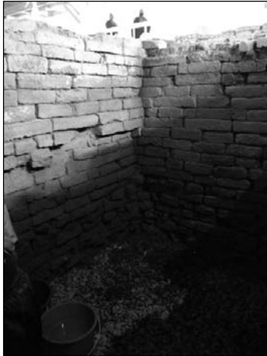
Figure 156. Degradation of the bricks in Trench C7
