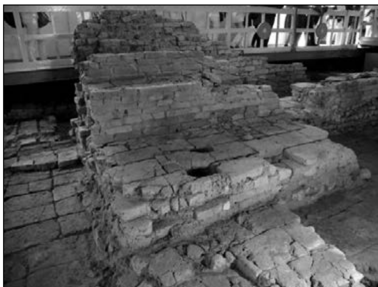
Figure 160. The South wall after the cleaning
