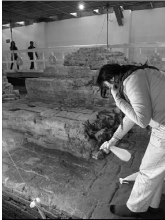
Figure 163. Spraying the final waterproofing/strengthening mixture
