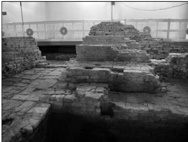
Figure 164. The South wall at the end of the restoration
