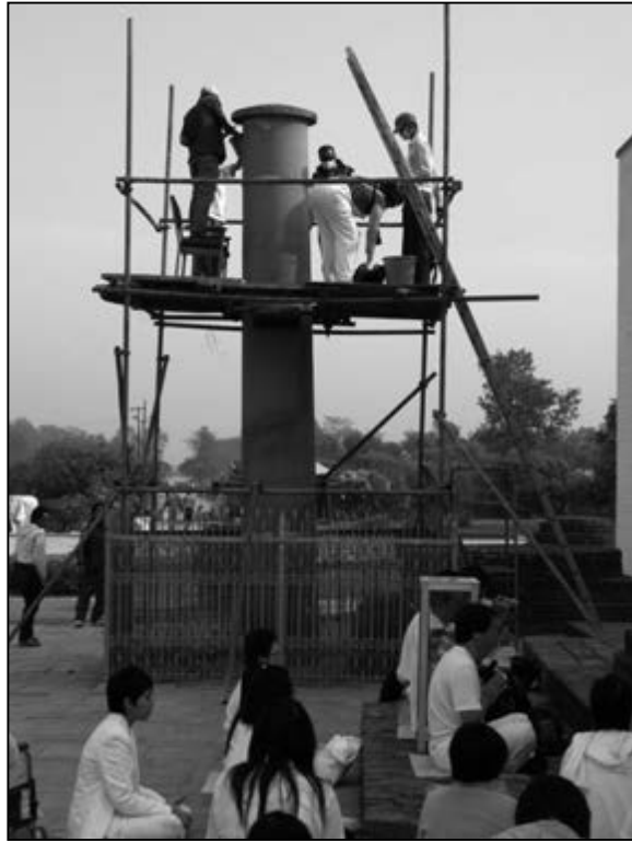
Figure 113. Scaffolding around the Asokan Pillar during the restoration work
