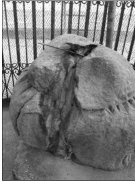
Figure 141. The two elements of the capital are connected with cement concrete
