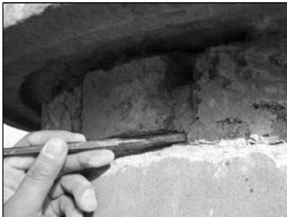
Figure 130. Mechanical removal of the cement mortar
