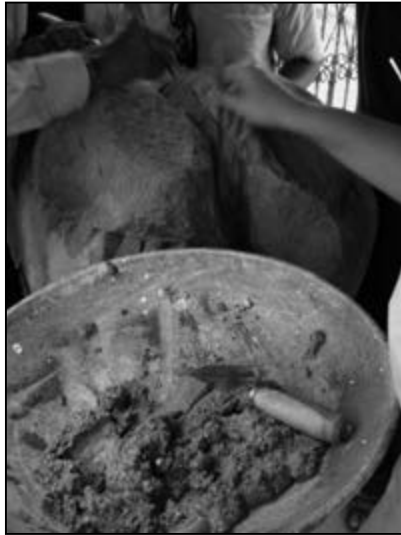
Figure 147. Filling the fissure with mortar.
