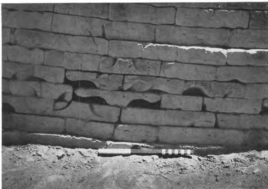
B. Paisia: Close-up of south face of temple No. 1, showing use of moulded bricks of earlier temple (No. 4) in the foundation
